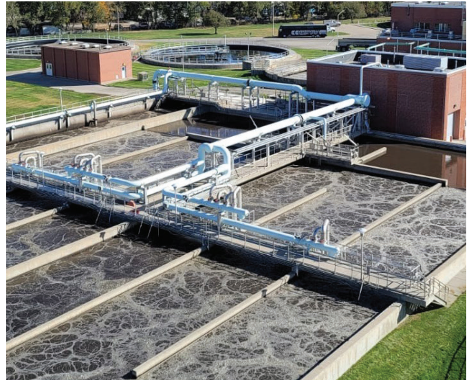
Activated Sludge Aeration Tanks
