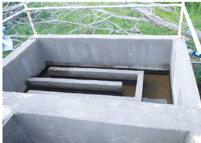
Chlorine Contact Tank
