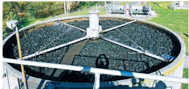
Trickling Filter
