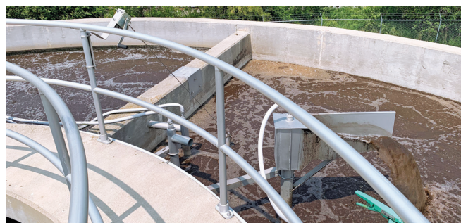
Aerobic Sludge Digester
