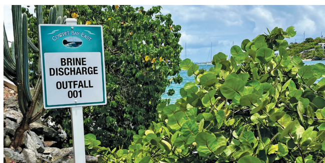
Effluent Discharge Point (also known as "Outfall")
