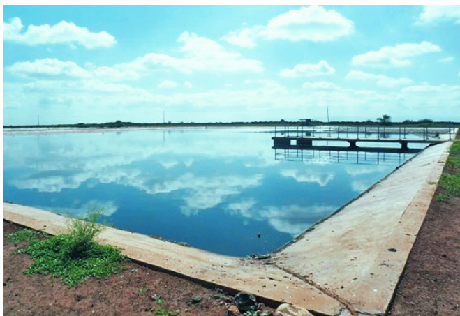
Figure 1. Facultative Lagoon. (Source: Water & Wastewater: Your Source for Water Clarity, 2024).
