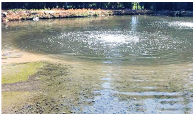
Figure 13. Figure 13. Sludge Accumulation. Photo Courtesy of Mark Cubbon. RCAC
