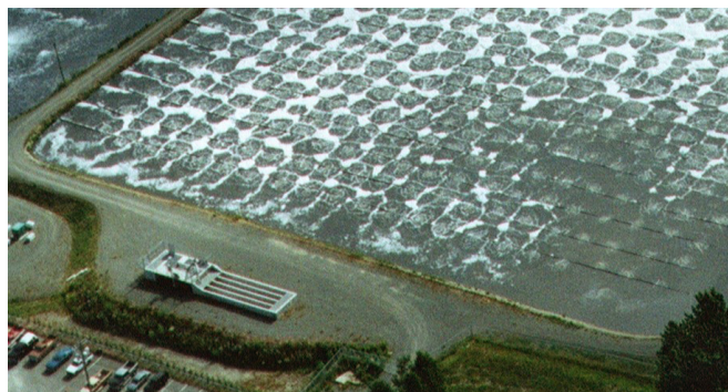
Figure 8. Diffused Aeration. http://northcowichan.bc.ca
