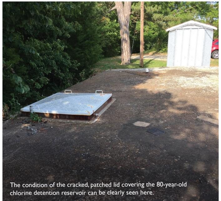
The condition of the cracked, patched lid covering the 80-year-old chlorine detention reservoir can be clearly seen here.
