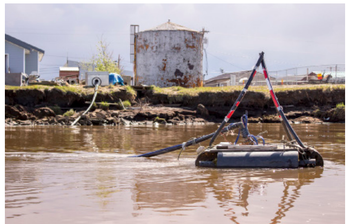
Water intake pump for the entire community (notice the bank erosion)
